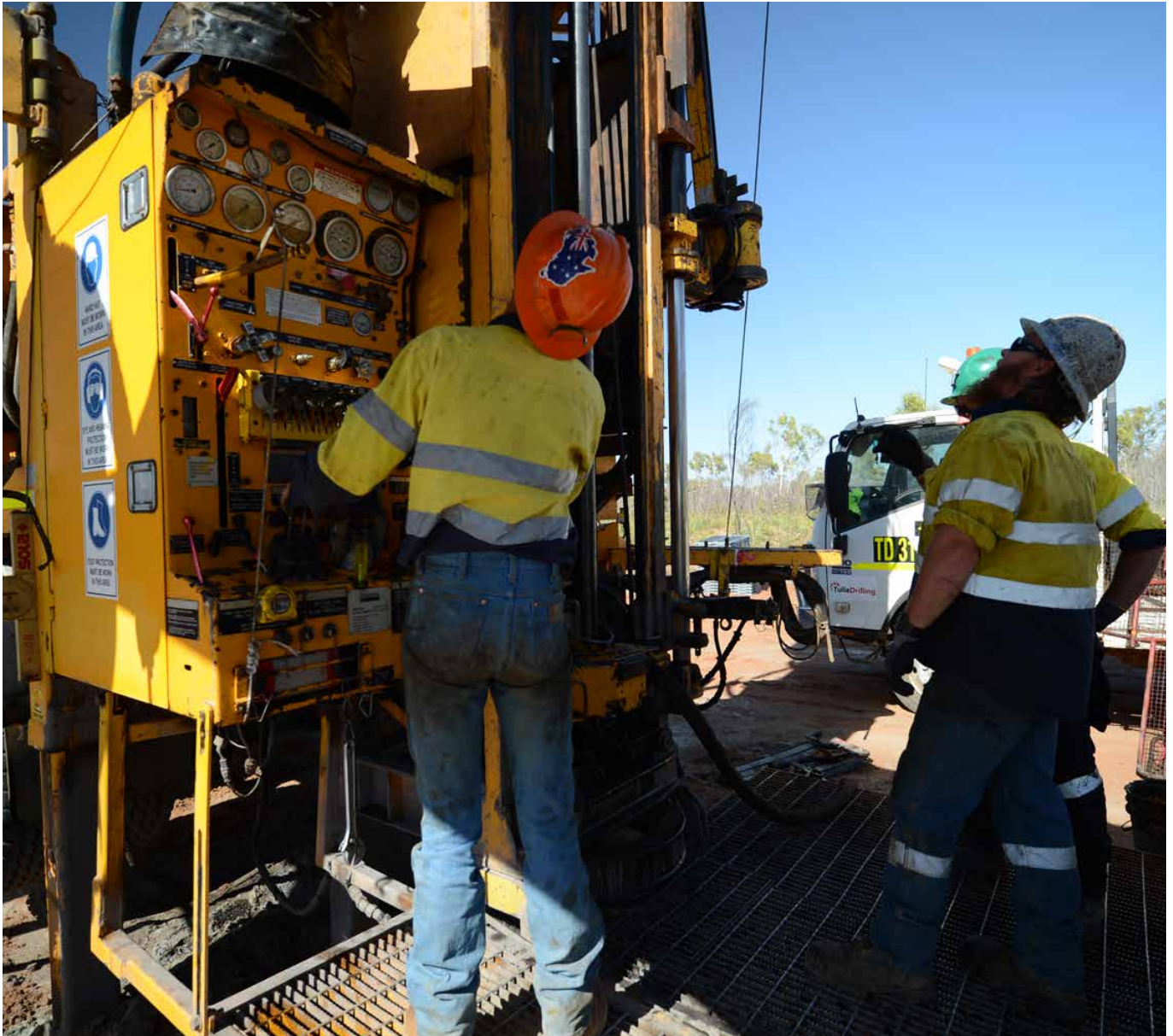
Figure 8: Exploration drilling at Superior's Greenvale Project
